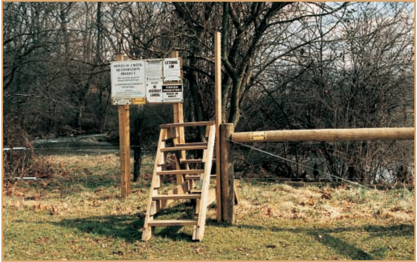
A constructed sign board informs the general public of acceptable conduct. A fence stile provides easy access over the stream-bank fencing.
