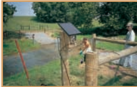
12 volt solar charger powers streambank fencing. Notice cattle-crossing in background.
