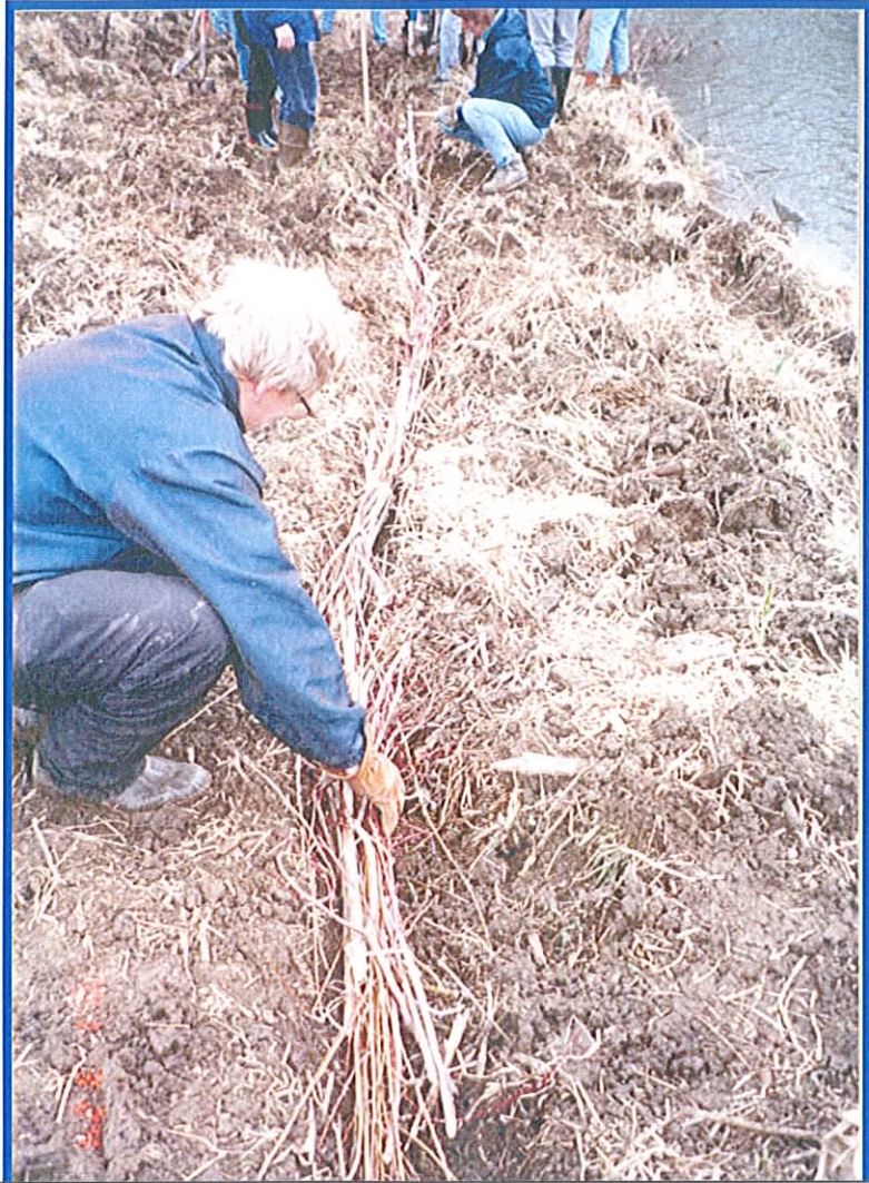
Fascine installation at Maple Grove – A “bioengineering” technique
